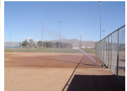
New Infield Irrigation at James Woody Park
