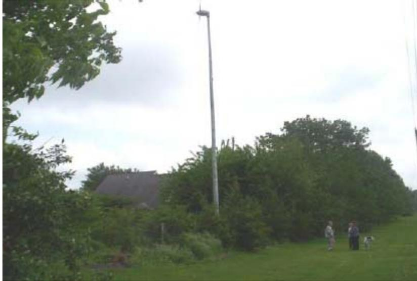
**5 kw turbine** – The 5 kw turbine shown in the picture below is on a sixty-four (64) foot tall tower with guy wires and a blade diameter of eighteen (18) feet. If the turbine operates at its maximum efficiency, it will generate over half of the annual electrical usage of a single family home. These turbines are designed for commercial or agricultural uses.
