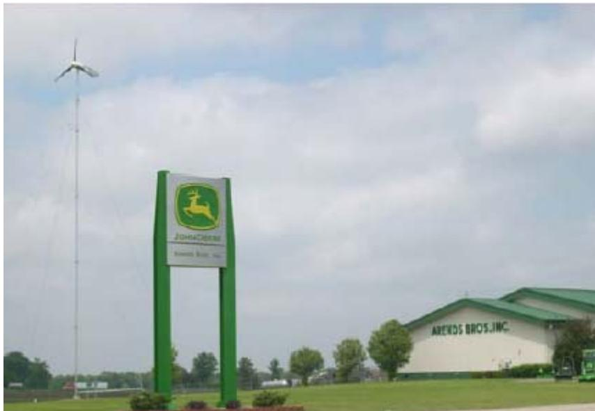
**10 kw turbine-** the 10 kw turbine shown below has blades with a twenty-two (22) foot diameter. This turbine is mounted on a 100 ft. lattice tower with guy wires. A 10 kilo-watt tower will typically generate enough energy to power a single family home. These are typically used for agricultural properties.
